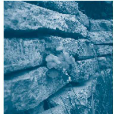
Recycled concrete wall (urbanite).
