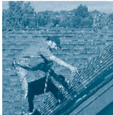
Installing Solar Water System
