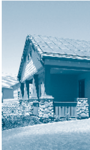
Photovoltaic System, Centex Homes, Livermore, CA
